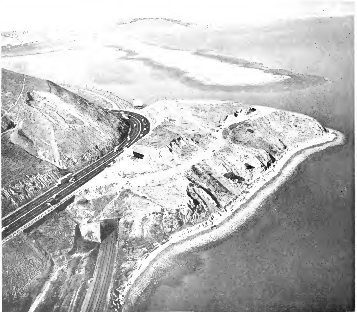
View of open water section of fill for Boyshore Freeway across Condlestick Cove, Sierra Point in foreground. Both railroad and highway will be relocated across the Point to the right of existing facilities. Purpose of railroad relocation is to provide additional tracks. Freeway will be carried over railroad on structure on solid ground at Sierra Point.
